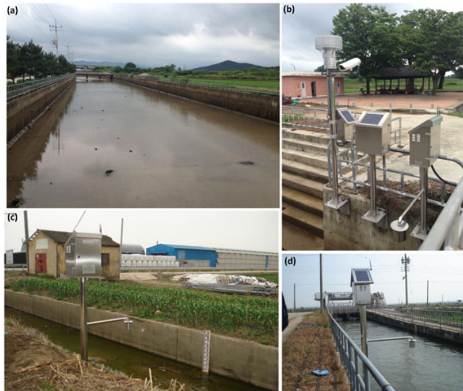
Figure 4. Automatic water level meters: (a) Gimjae open main canal, (b) Gimjae secondary inlet canal, (c) Jongshin secondary outlet canal, and (d) Jinbong secondary inlet canal
